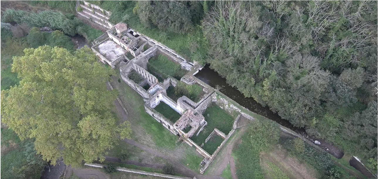
Fig. 3. The complex of the «Mulino-Ferriera Alviggi» in a top view from drone (photography by the author).
