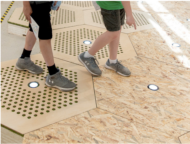
Fig. 9. The Dynamic Street (image credits: David Pike). In collaboration with Alphabet's Sidewalk Labs, CRA developed The Dynamic Street , a prototype of a modular and reconfigurable paving system hinting at the possibility of the future streetscape seamlessly adapting to people's needs.
