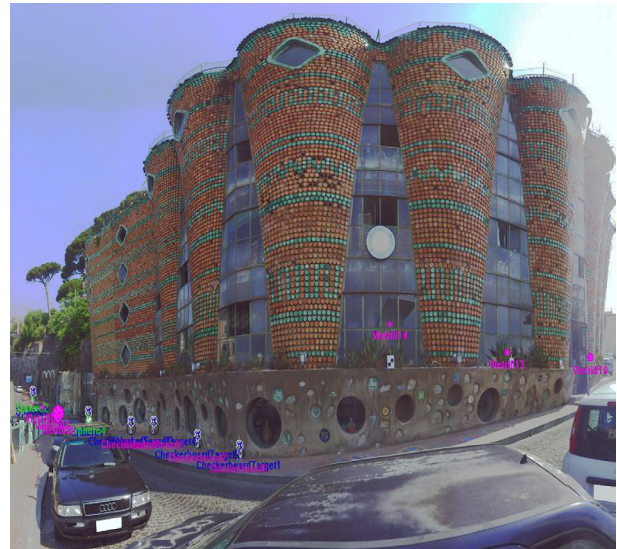
Fig. 4. Location of targets and survey station points.
