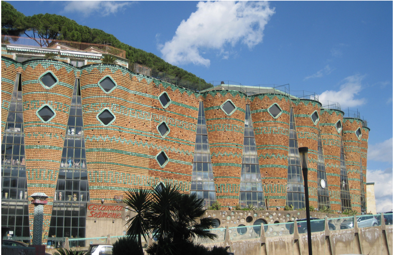
Fig. 1. South front of the Solimene factory (photo by the authors).
