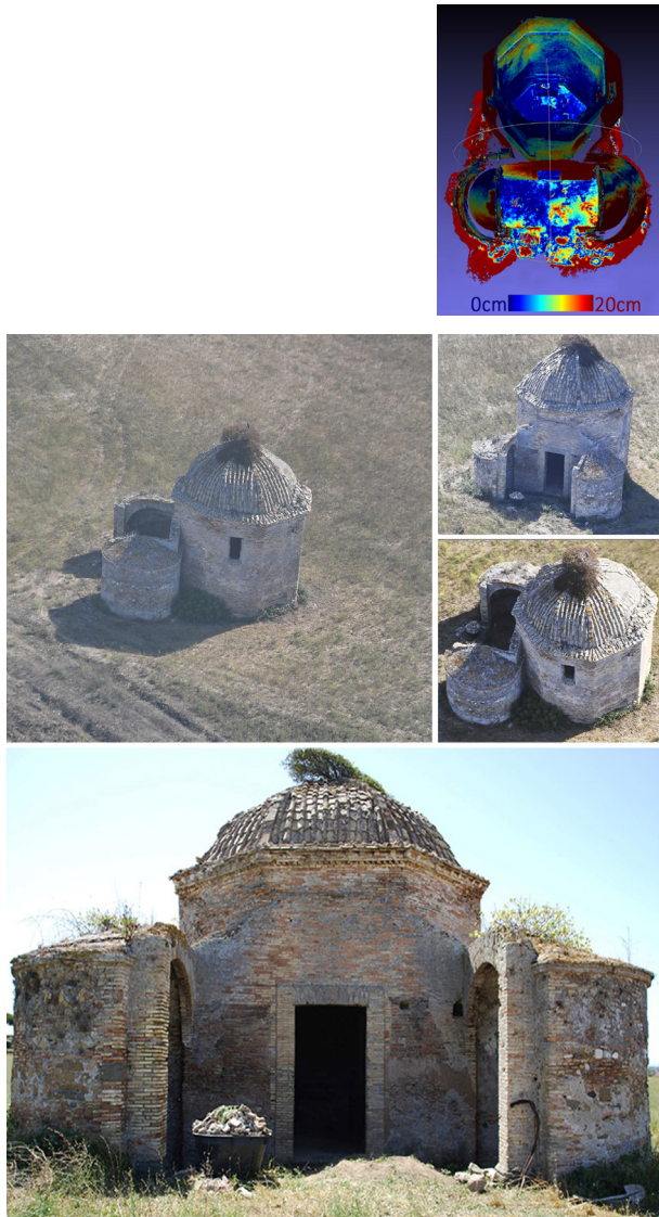
Fig. 3. Church Santa Maria delle Vigne in Pratica di Mare, Rome. Photo of the current state and point cloud obtained by a survey made with the Tango technology
