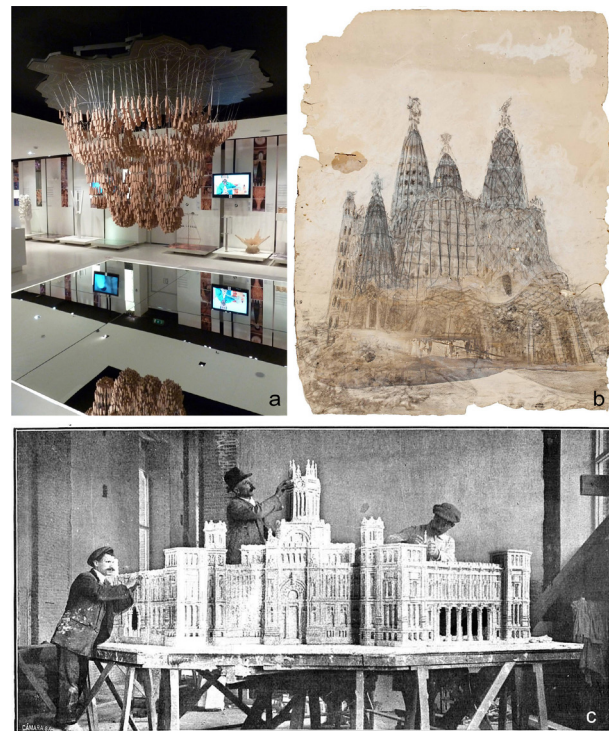
Fig. 7. a) Reconstruction of Gaudí’s structural model for the church (not built) of the crypt in Park Güell (Barcelona), displayed in the Gaudí Centre in Reus (Tarragona). In the lower mirror, you can see the final form the building would have had (photo by the author, 2010); b) sketch of the exterior of the Church of Colònia Güell, by Gaudí (1898-1908); c) plaster model of the “Palace of Communications” in Madrid, work of Antonio Palacios. Mundo gráfico , Year II, No. 35, 26 June 1912.
