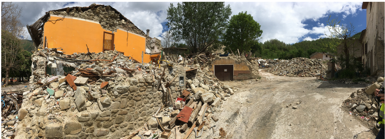
Fig. 1. Municipality of Accumoli, borough of Grisciano after the removal of earthquake ruins.
