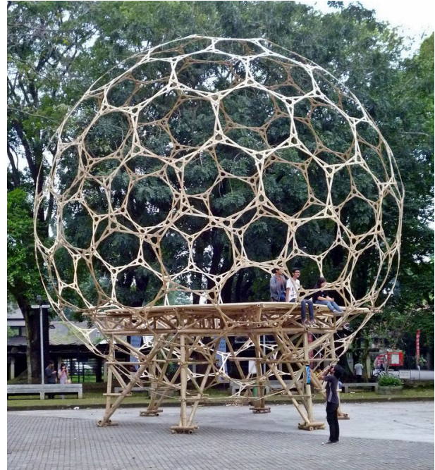
Fig. 6 Prof. Bando Takaaki collaborative project to make bamboo shelter that shapes in inspired by Buckminster Fuller's dome [Larasati 2012] < https://investor.id/property/32710/takaaki-bando-jadikan-bambu-hunian-masa-depan > (accessed 2025, October 21)
