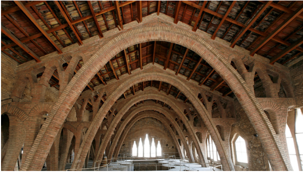
Fig. 1. Detail of the main beam of the Pinell de Brai Cooperative, built with brick arches. Image credit: Department of Culture of the Generalitat de Catalunya.
