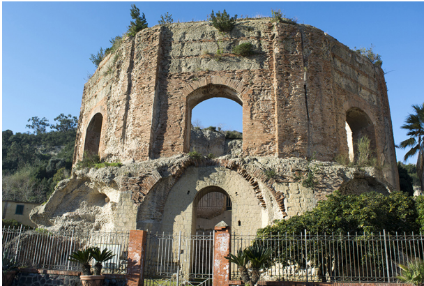
Fig. 2. View of the surviving portion of the dome and the openings in the drum (photograph by S. Bertacchi).
