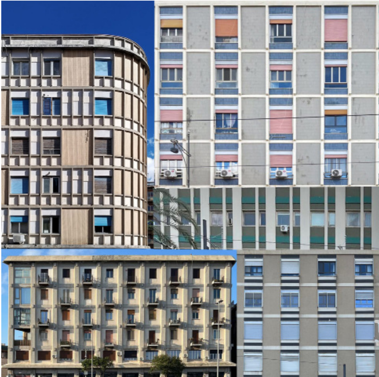
Fig. 5. Buildings with facades defined by coplanar structural elements (photos by the author).
