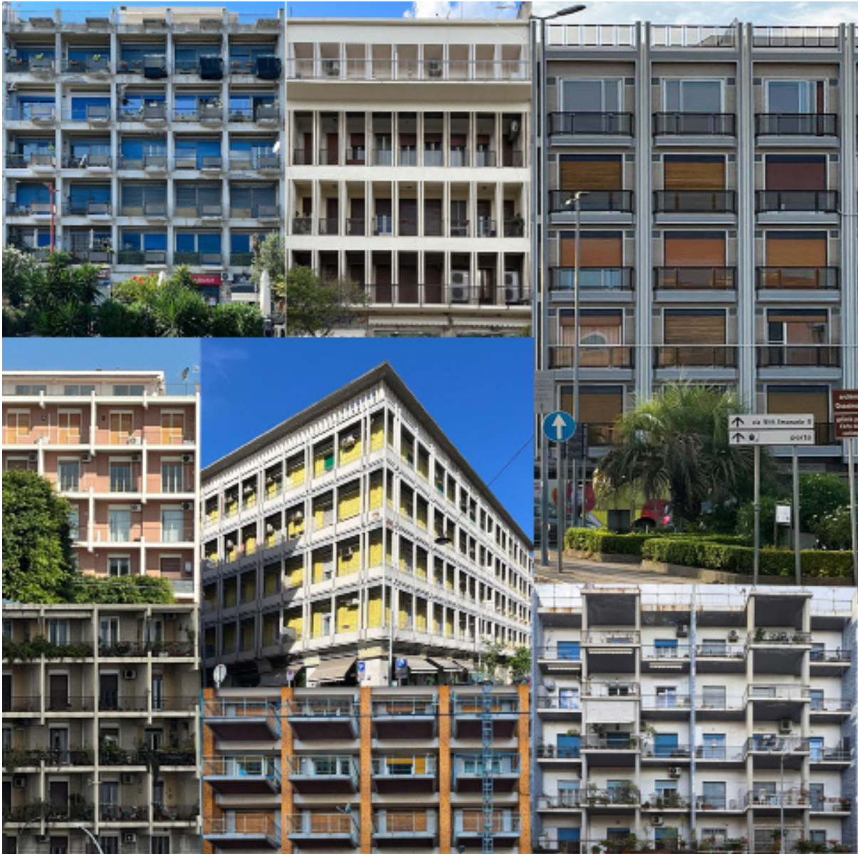
Fig. 7. Buildings with facades defined by structural elements external to the facade (photos by the author).
