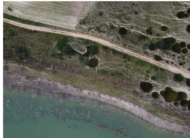
Fig. 5. Aerial view of the fourth bunker belonging to the "Licata" and located near the shore of Simbirizzi Lake (photo by Nicola Paba).
