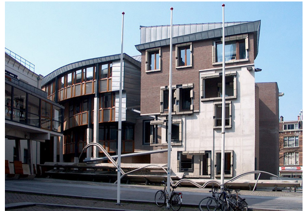
Fig. 10. Enric Miralles and Benedetta Tagliabue, Extension of Utrecht Civic Hall, 1997-2000 (photo by the author).
