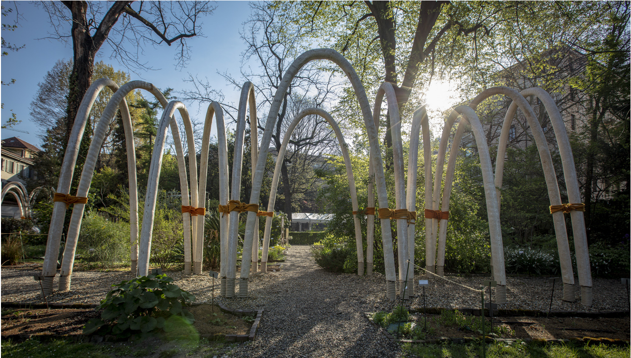
Fig. 13. The Circular Garden (Image credits: Marco Beck Peccoz). For Fuorisalone 2019, a part of Milan Design Week, CRA, in partnership with global energy company Eni, developed an architectural structure made of mycelium, the fibrous root of mushroom.
