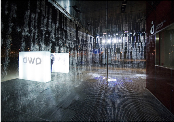
Fig. 1. Digital Water Pavilion (image credits: Claudio Bonicco). The Digital Water Pavilion, made for the 2008 World Expo in Zaragoza, Spain. The design teams at the MIT Senseable City Lab and Carlo Ratti Associati (CRA) created a reconfigurable space, with walls composed of digitally-controlled water droplets.
