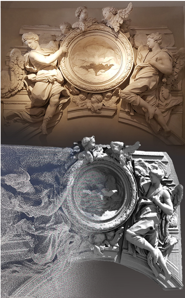
Fig. 4. Sculptures above the niche on the left side in the nave of the church of the Stimate : photo and laser scanning survey.
