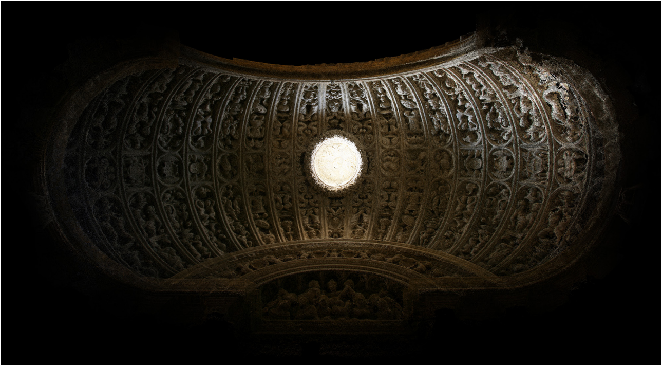
Fig. 1. Point cloud of Capilla de Junterón's vault obtained with the laser scanner Faro Cam2 (rendering by A. Bortot).
