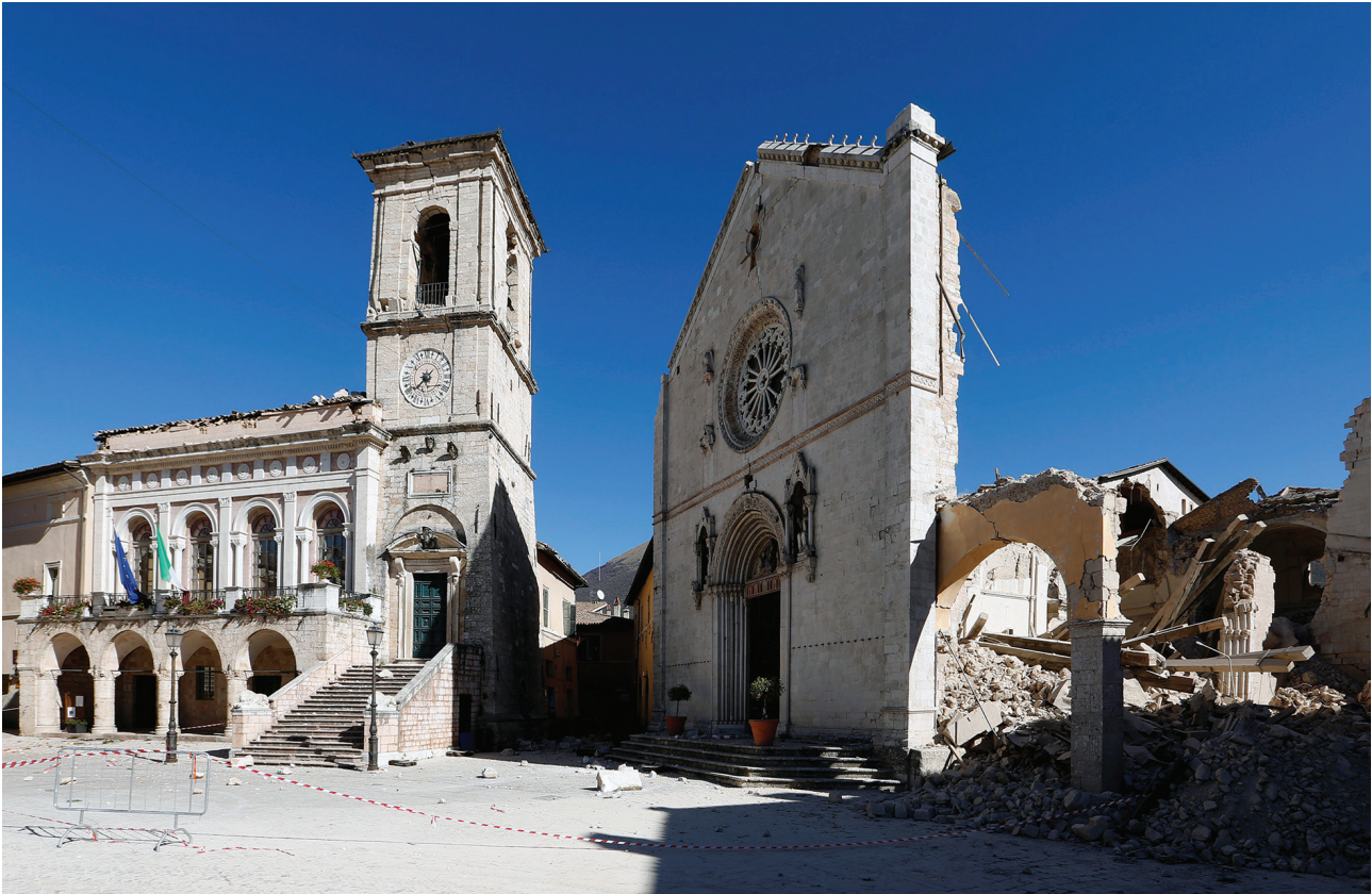
Fig. 1. Norcia (PG), the Basilica of San Benedetto after the earthquake of 30 October 2016.
