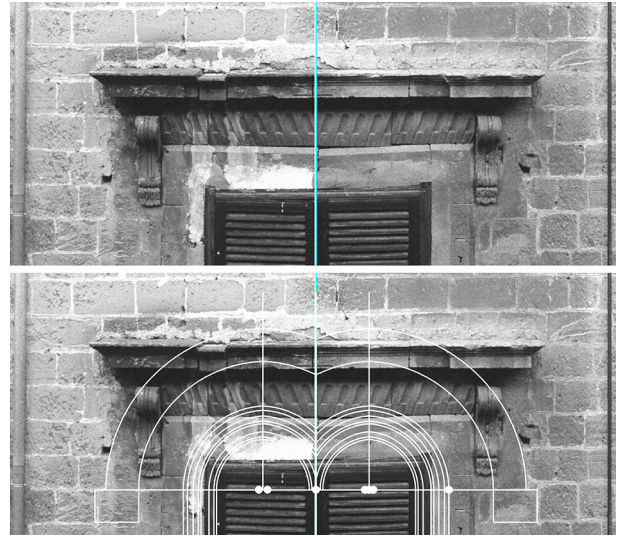
Fig. 7. Traces of the double-arched window 7 at the piano nobile.
